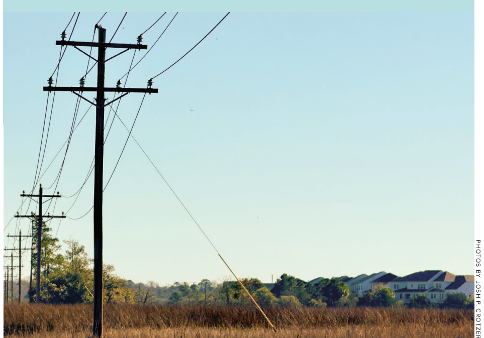
Berkeley Electric's overhead lines stand among the marsh near the Stono River. These lines are slated to be converted to steel poles to improve reliability for this booming community.
