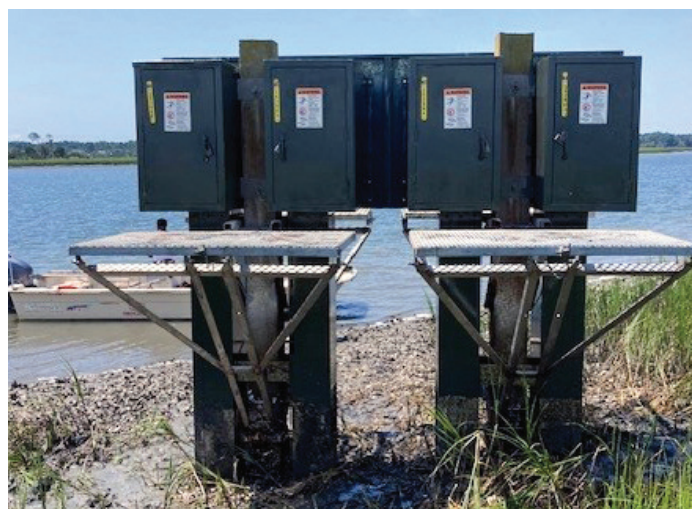
Accessible only by boat, these electrical cabinets serving an underwater cable crossing the Stono River needed to have the platforms replaced due to saltwater corrosion.
