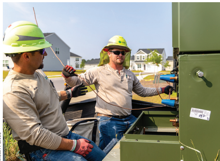
Linemen Kyle Childers (left) and Ashby Freeman prep one of several underground transformers that will serve a new subdivision in Carnes Crossroads.
