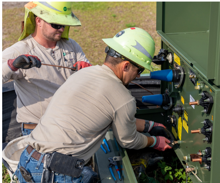
Linemen Ashby Freeman (L) and Kyle Childers set underground transformers in Hewing Farms, a new residential development in Carnes Crossroads. Strong residential growth is adding 5,000-7,000 meters to the co-ops system annually.
